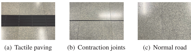
Fig. 7: Examples of tactile paving, contraction joints, and a normal road.
