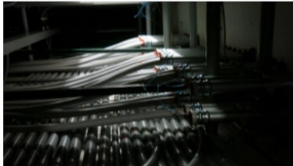
**Figure 4** The design choice to use pre-assembled cabling (TC Cable, as pictured) instead of in-house assembled cabling to provide the 24,000 linear feet of electrical cable required to connect Trinity resulted in an estimated \$1M project cost savings.
